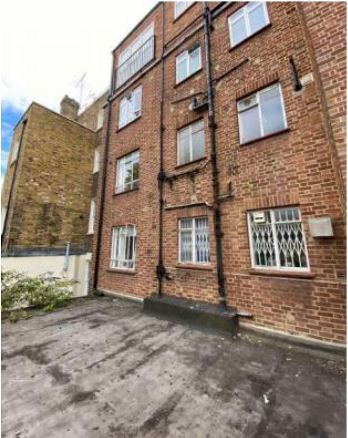
View looking to the rear elevation (location of proposed terrace)
