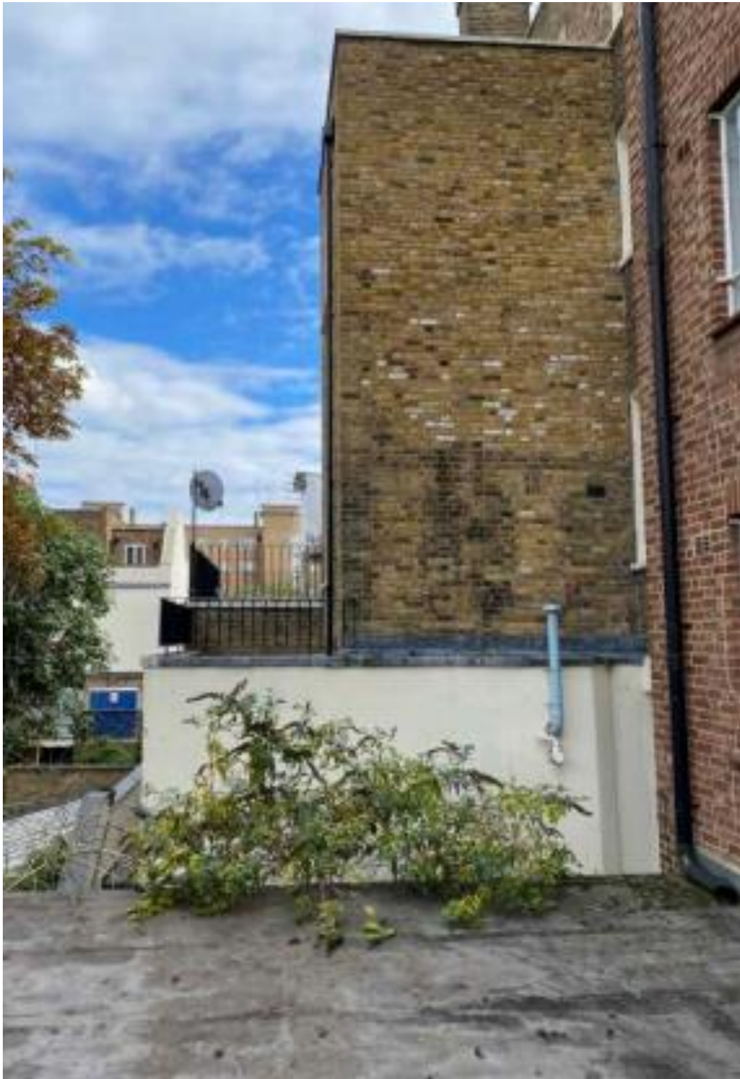
View looking to the south of the site
